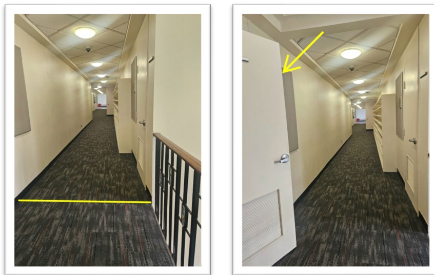
Figure 6: Images of Egress Location; Yellow line indicates location of new wall, yellow arrow indicates door to be closed in (Not picture in floor plan).
